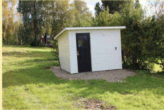
The pump house (9 m<sup>2</sup>) is built of concrete blocks with a face of wood, has two floors which one is under the surface.
